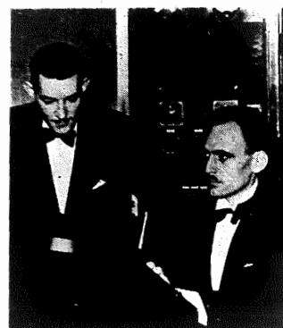
CBS Control Room in Detroit
